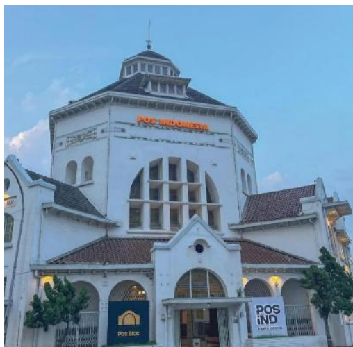
Figure 1.0 Front view of Medan Post Office (Post Bloc)
